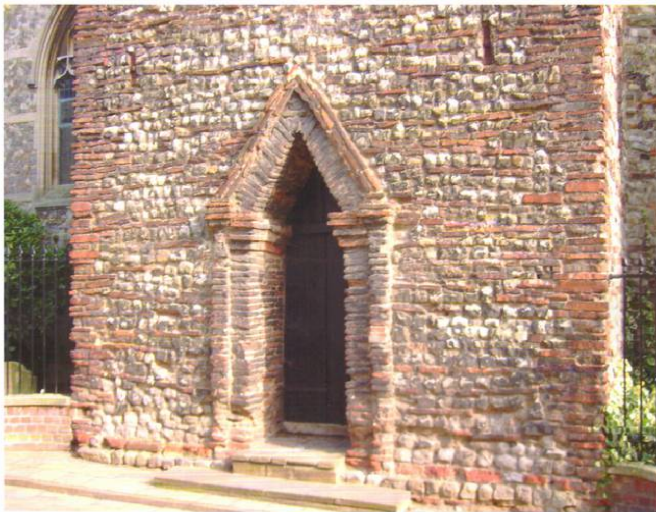
Roman building materials were still readily to hand when the doorway to Holy Trinity church was constructed in the centro of Colchester, possibly around 1050 AD
